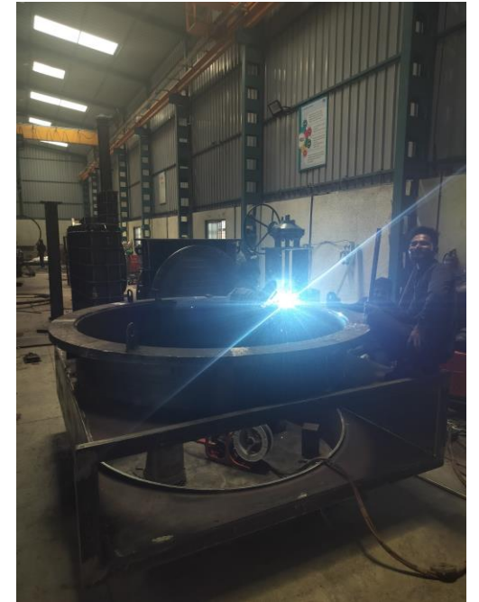
WELDING IN PROGRESS
