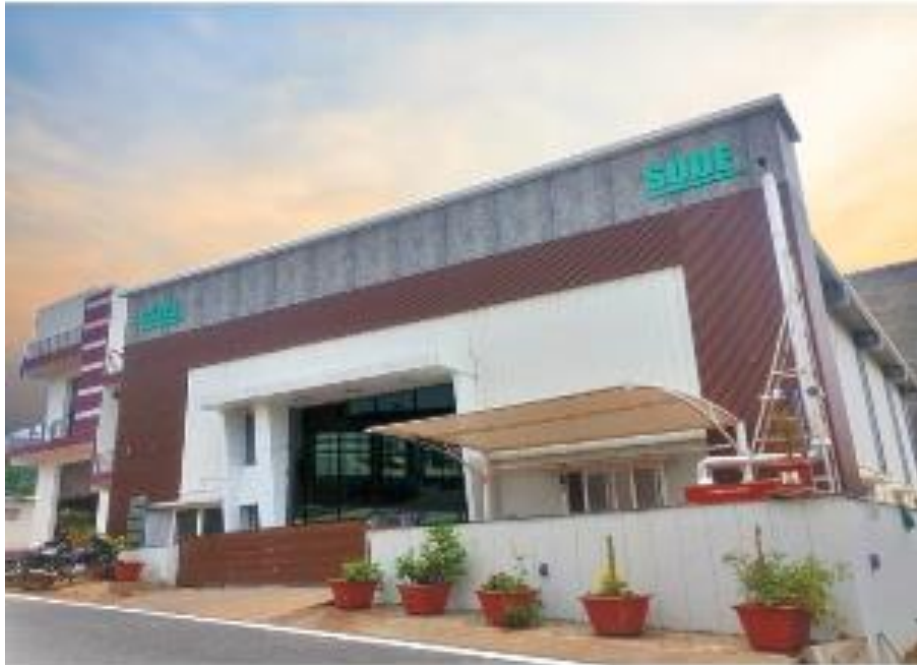
Office & Works - Bangalore
